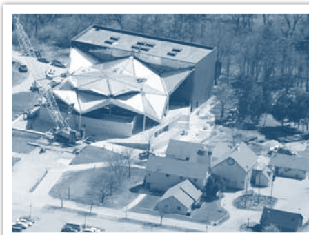
The Starlight Theatre's Bengt Sjoström Theatre (BST) was transformed (between 2001-2003) architecturally with a design by Jeanne Gang Associates. The construction and design resulted in international
